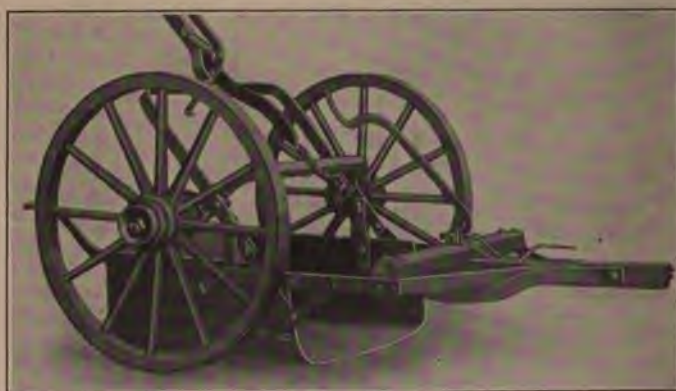
Wheel Scraper, ready to Load.
